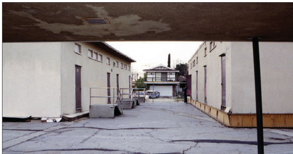
Figure 4-7: Modular classrooms pushed off their foundations; note stairs at left, Northridge, CA, 1994
